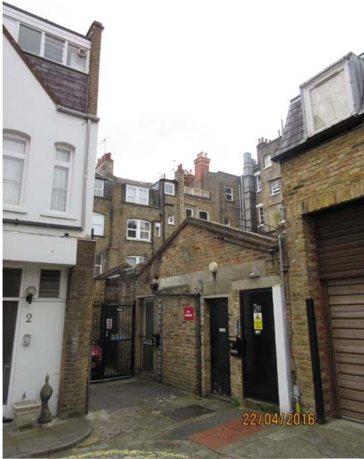
View of the site from Charles Lane
